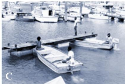
Fig 4 – Stages in construction and installation of marina. – (a) pile driving (1983); (b) Fabricating GRC-covered polystyrene blocks for floatation units at Hornibrook Steel; (c) Manoeuvring an 11-metre walkway into position.
